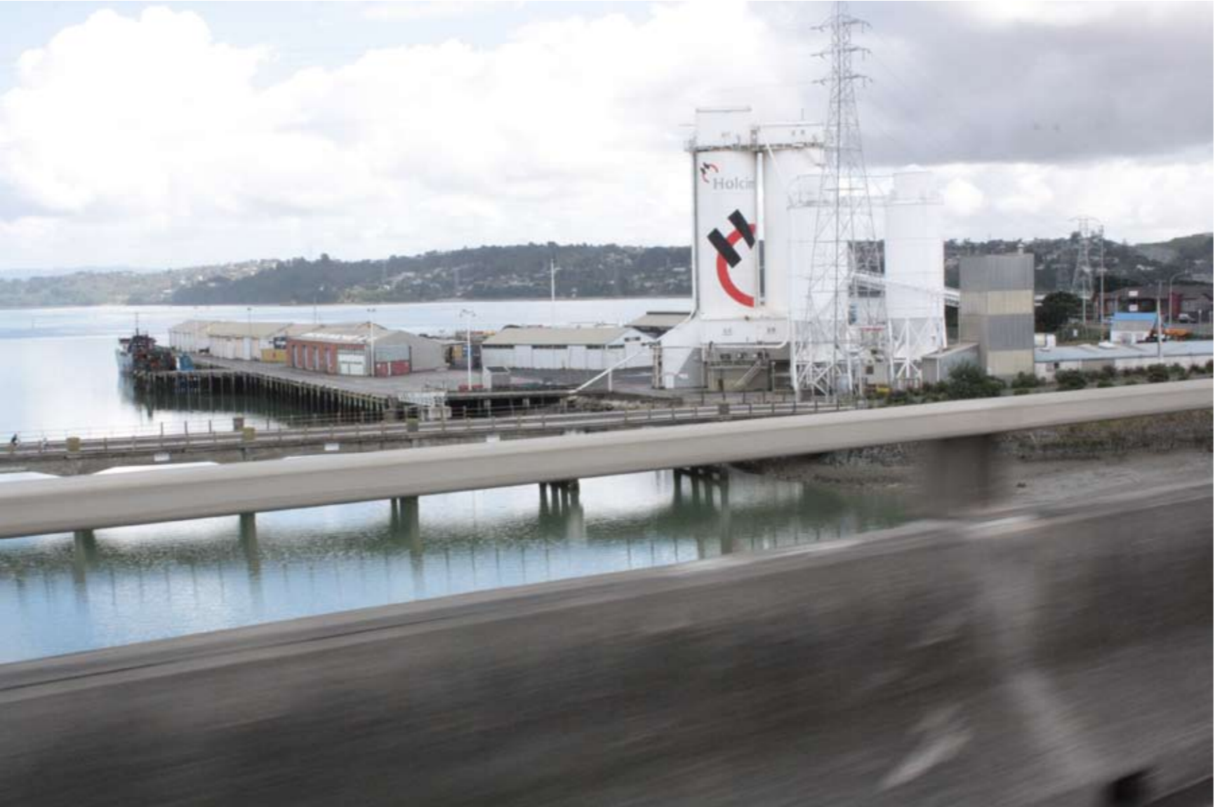
View from Mangere Motorway Bridge
